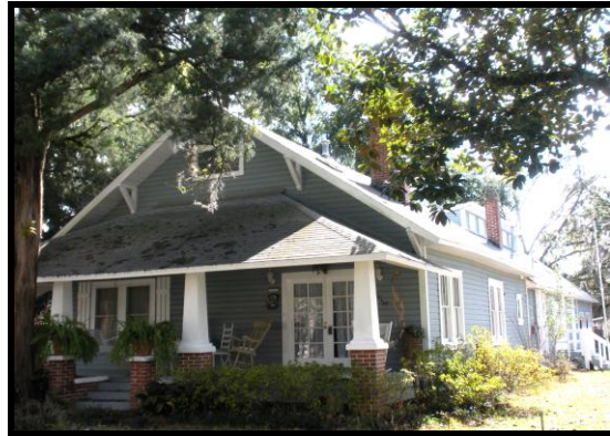
Figure 30. 25467 SW 1 st Avenue (8AL2405)
